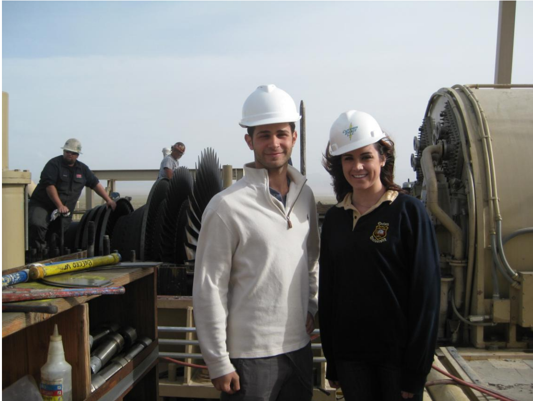
Dixie Valley Geothermal Power Plant
