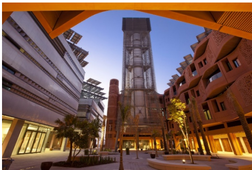
Figure 7 Wind Tower and Central Courtyard. Photo from Masdar Official. Licensed by CC BY-NC-SA 2.0
