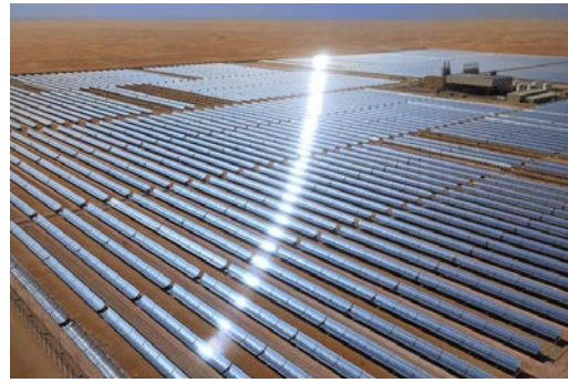
Figure 1: SHAMS 1 Concentrated Solar Power Plant. 256,048 Mirrors in an area of 2.5 km 2 . Licensed by CC BY-NC-SA 2.0.
