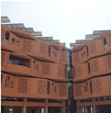
Figure 4: Facade of the Masdar Institute Dormitories. By Masdar Official. Licensed by CC BY-NC-SA.
